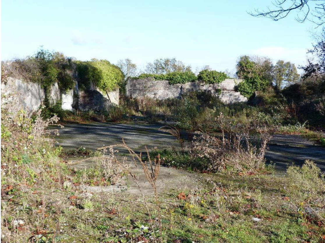
Plate 11.11: Remaining walls of house and outbuildings, 'Belcamp'.
