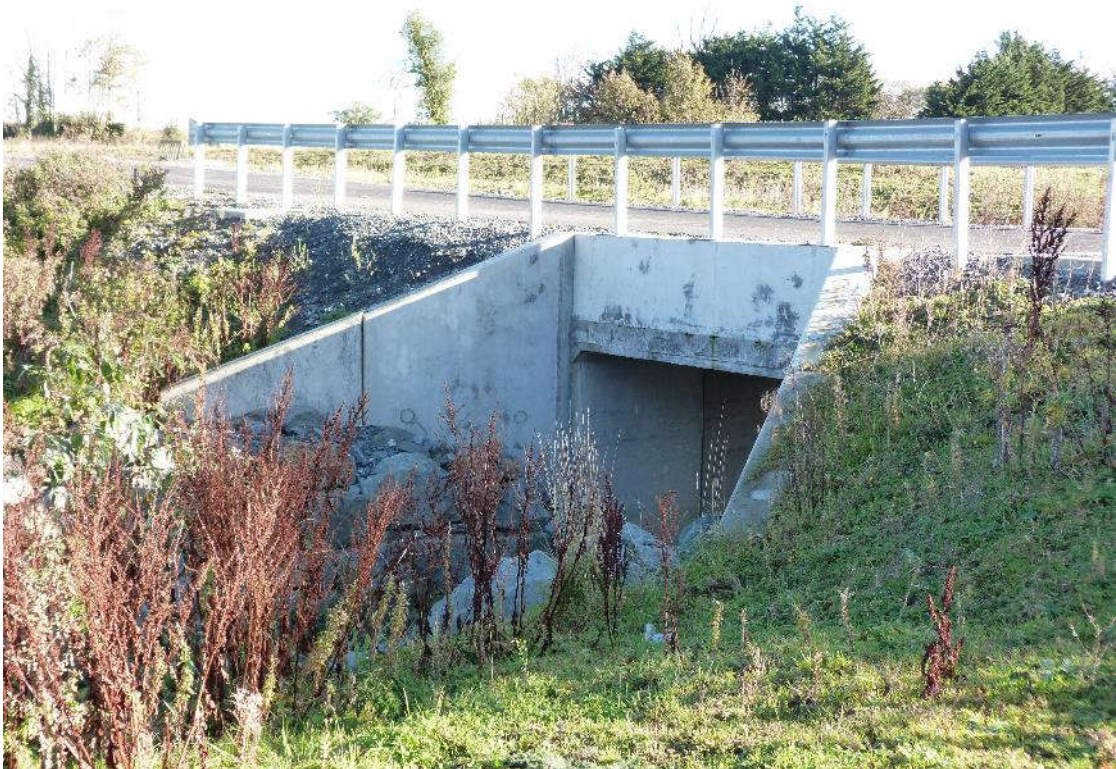
Plate 11.10: Modern concrete bridge and access road over River Mayne.
